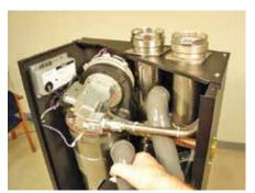
Removing combustion air intake riser
