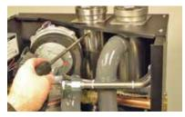
Flue gas test port plug
