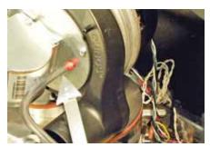
Fan pressure sensing tube
