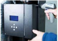
Removing wiring box covers
