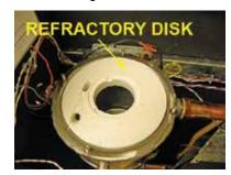
Combustion Chamber Refractory
