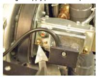
Manifold pressure test port
