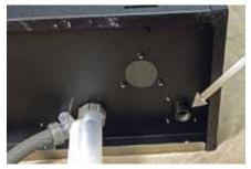
Gas inlet connection on bottom
