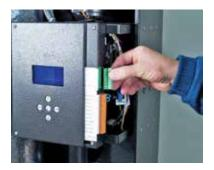
Line voltage load pump terminals
