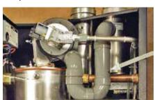
Combustion air intake riser
