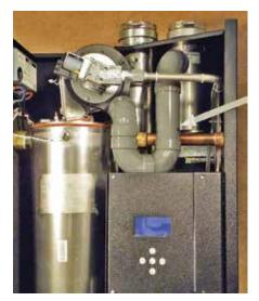
Combustion air intake riser
