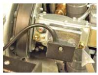
Inlet gas supply pressure test port
