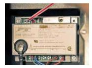
Fenwal ignition module -Microamp (µA) test points are shown at top left corner of module (beside red L.E.D.)
